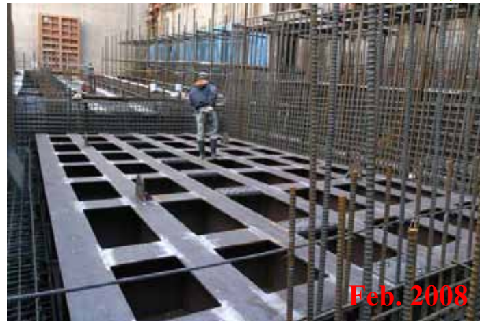
Anchor frame for BD core
