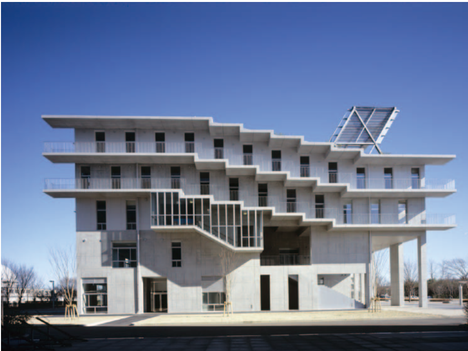
A spiral structure of the IPMU building can be clearly seen from this side. Photo: Toshiharu Kitajima
