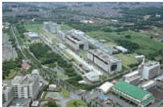
■ Figure 3: Aerial view of the Kashiwa campus.
