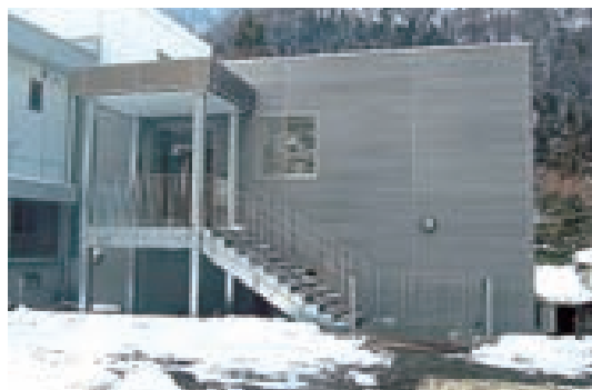
■ Figure 5: The Kamioka Satellite Office building.
