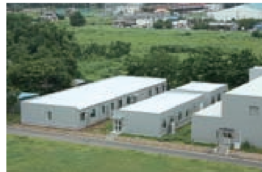
■ Figure 4: IPMU temporary buildings.
