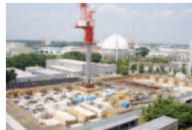
Fig. 2 Construction area of the General Research Laboratory Building.
