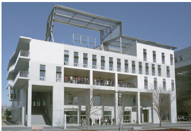
The IPMU Research Building
