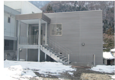
Kamioka Satellite Research Building
