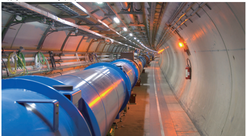
Figure 4. The first LHC magnets to be installed in the LHC tunnel. Copyright © CERN, Photograph by Maximilien Brice
