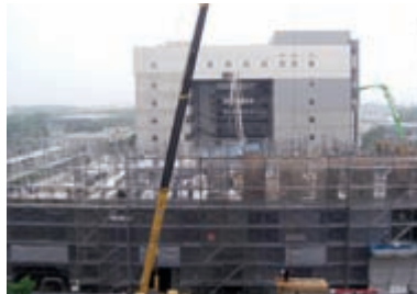
Construction area of the IPMU Research Building as of June 10
