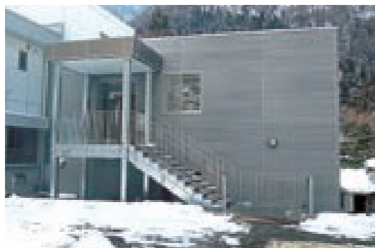
■ Figure 5: The Kamioka Satellite Office building.
