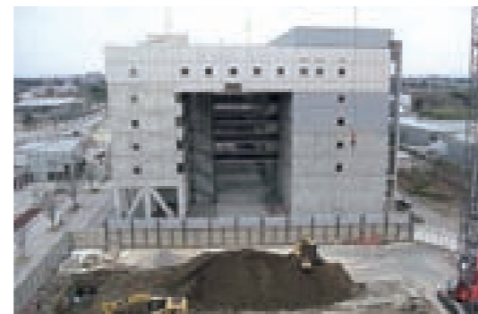
■ Figure 6: New laboratory under construction.
